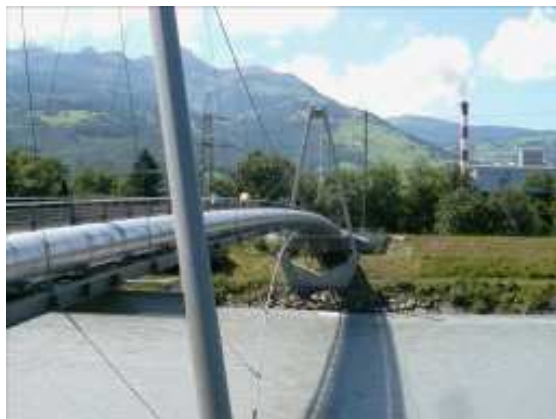
Figure 29: The new Energy Bridge across the Rhine, between the canton of St. Gallen and Liechtenstein, serves as a bicycle path and carries the steam pipe from the KVA (background, right). © M. Fasel
